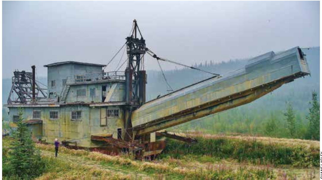
The Pedro dredge near the town of Chicken is a reminder of the rich placer gold in the streams of the Fortymile Mining District in eastern Alaska. In addition to gold, Doyon lands in this area host zinc, lead, silver, and copper.
